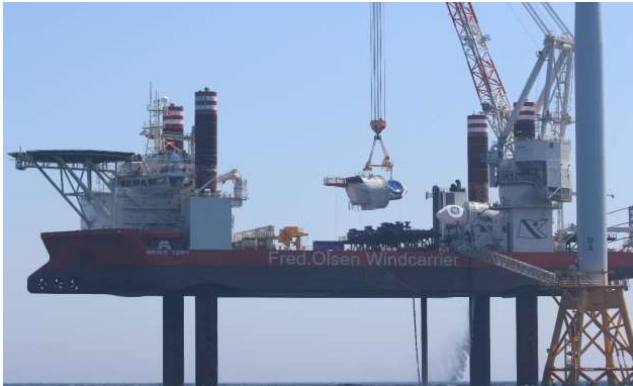
Figure 16. Lifting nacelle off the deck of L/B Brave Tern.
