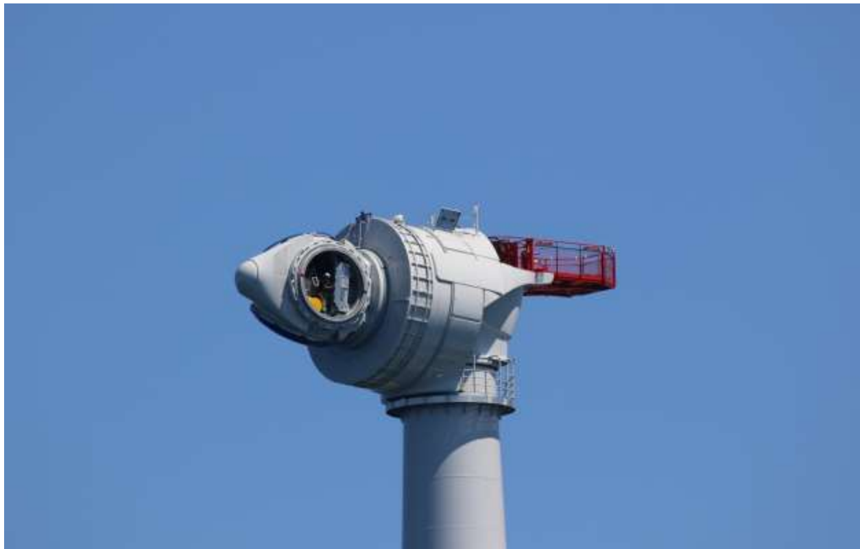
Figure 17. Nacelle placed on top of tower section.
