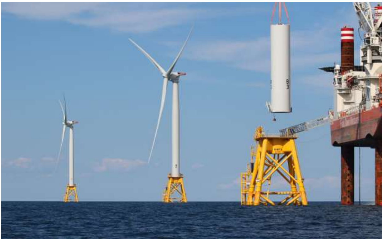
Figure 13. Close-up view of tower installation at WTG 3.
