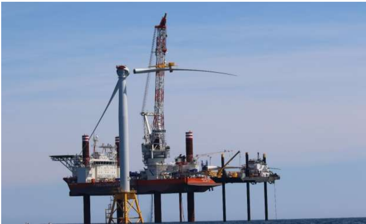
Figure 19. Attaching blade to nacelle at WTG 4.
