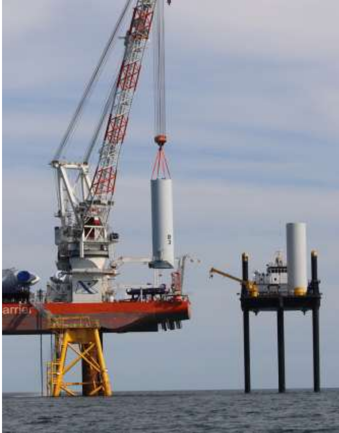
Figure 12. Placing the tower section at WTG 3.
