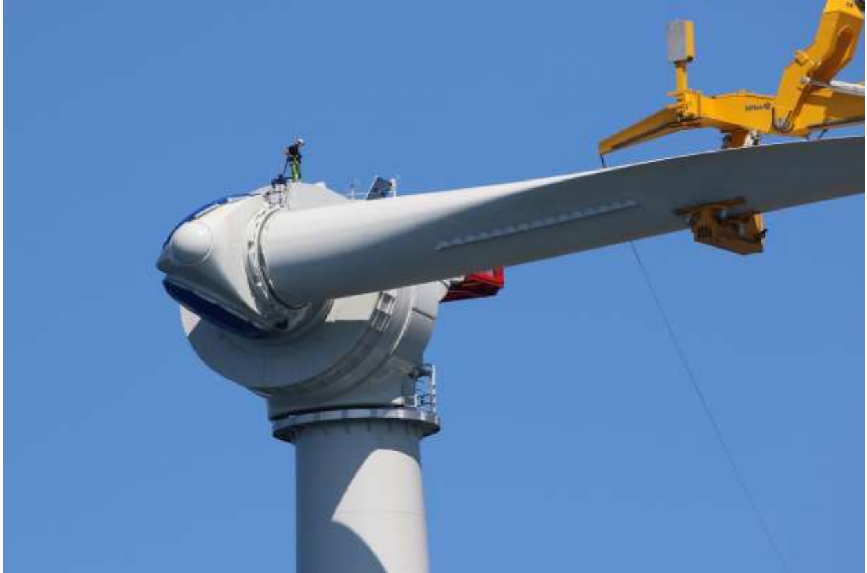
Figure 20. Worker securing blade to nacelle.
