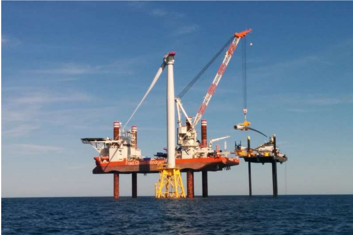
Figure 1-1 Jacket with four driven piles under construction
