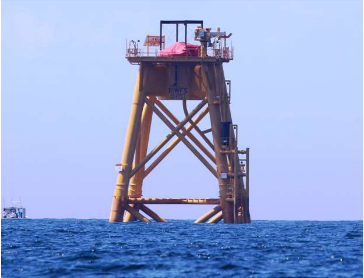
Figure 3. Fully assembled WTG 5 foundation
